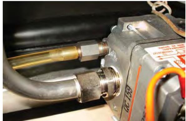
– Have installer follow gas pressure requirements. Installer should check incoming gas pressure and manifold pressure with all equipment in the kitchen on and operating.
